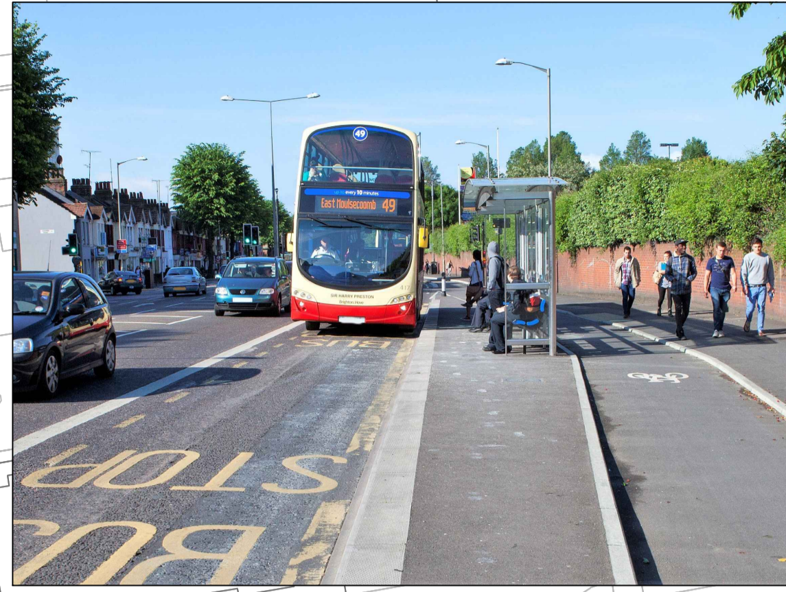
Image 2 - Example of floating bus stop
