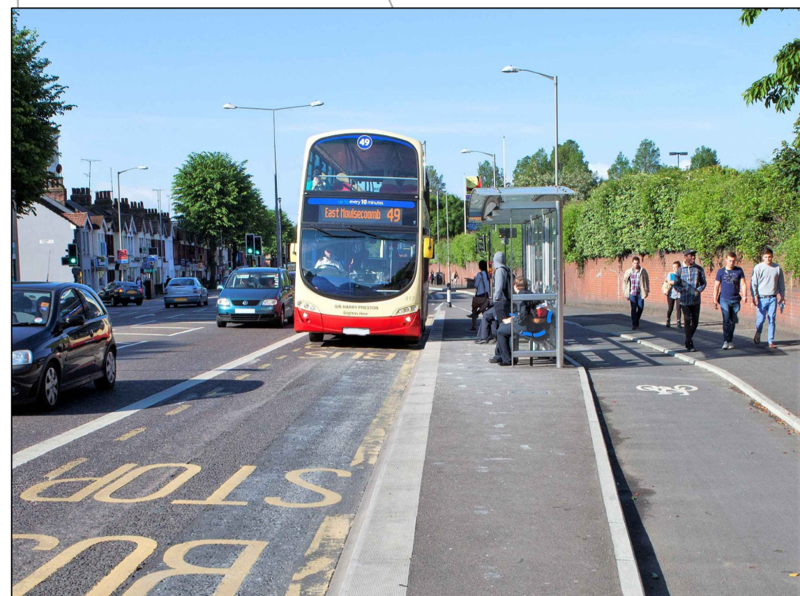
Image 2 - Example of floating bus stop
