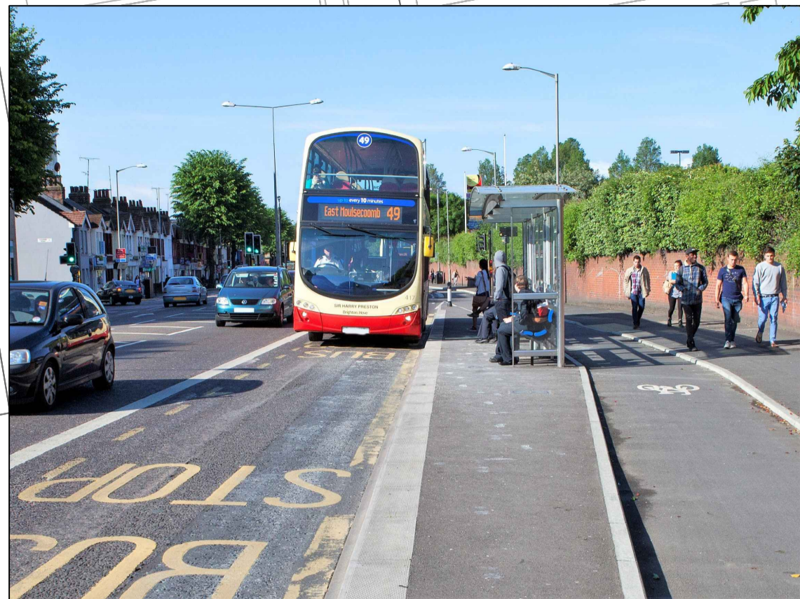
Image 2 - Example of floating bus stop
